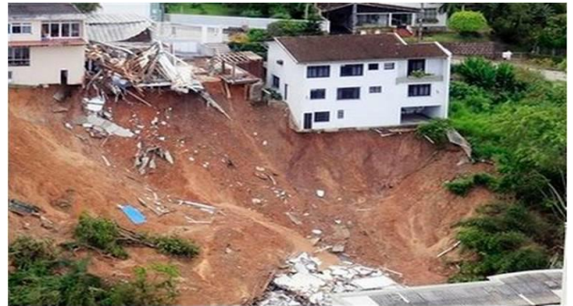
Figure 5: Landslide in Uttarakhand on a locality (2013).
